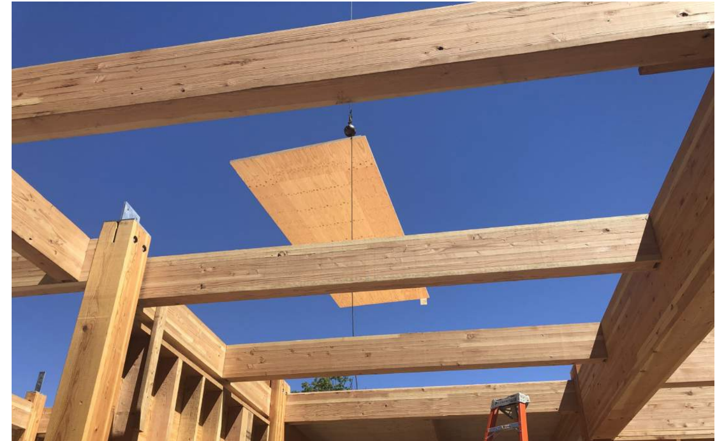
Photo: Bush School, Mass Ply Wood Panel (MPP) Installation; Mithun
